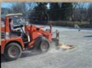
5 Filling joints and voids with rock chips.
