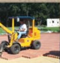
mechanical installation to earing course.
