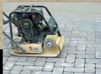
6 Compacting the permeable system.
